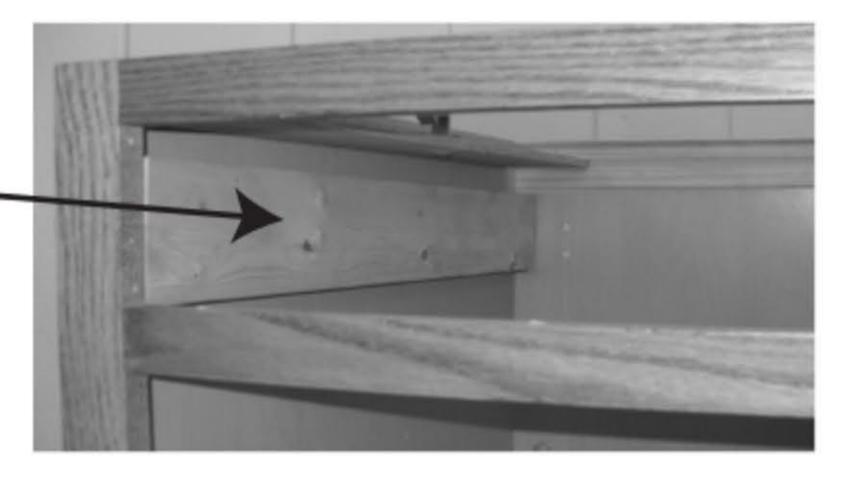
Step 3. Mark the location of the front mounting hole by measuring UP 1¾" from the LOWEST point of your opening and BACK ¼" from the front of the opening. Once marked install slides to side of cabinet insuring they are level.
